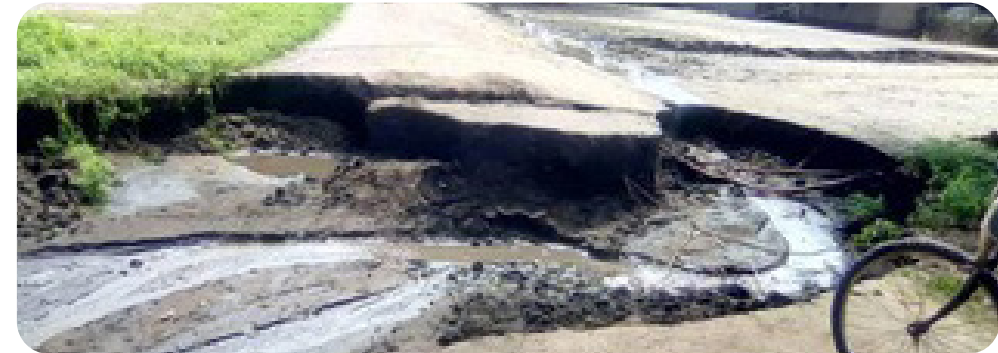
This is the road damaged by Cyclone Freddy, 1 kilometer from the Teen Missions base in Mangochi, Malawi. They are unable to drive in or out at this time.
